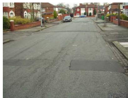
Photo's illustrating a range of amber1 and amber2 condition roads (includes need for surface dressing (1) and Micro Asphalt (2))
