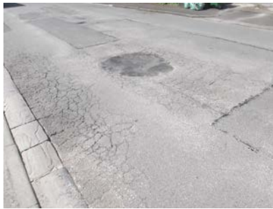
Photos illustrating a range of red condition roads (includes need for resurfacing (1) & reconstruction (2 & 3))
