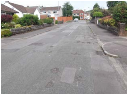
Photos illustrating a range of red condition roads (includes need for resurfacing (1) & reconstruction (2 & 3))
